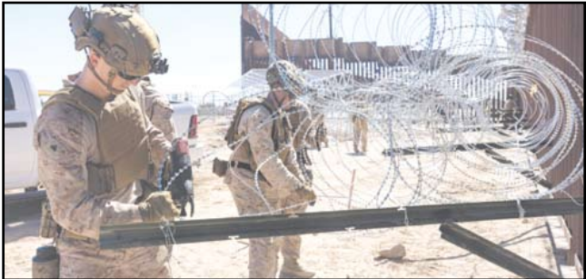
Marines Corps with 1st Marine Logistics Group, supporting Joint Task Force Southern Border, tie concertina wire onto a prefabricated bracket to reinforce the southern border barrier in Yuma, Ariz., July 29. U.S. Marine Corps photo by Sgt. Mary Torres
