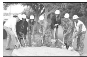
Groundbreaking for Child Development Center at Naval Base Point Loma May 10, 2024. U.S. Navy photo
